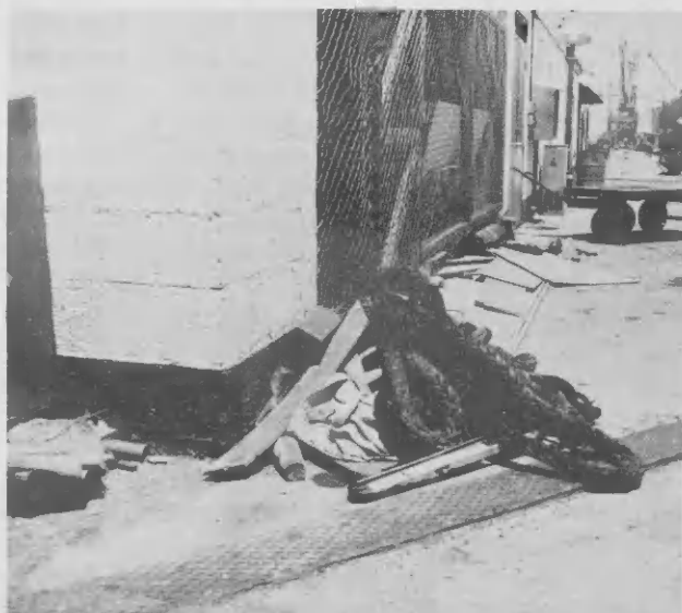
Another eye sore and unsafe situation: a1 Finger Pier # 2. Junk like this must be completely eliminated.
